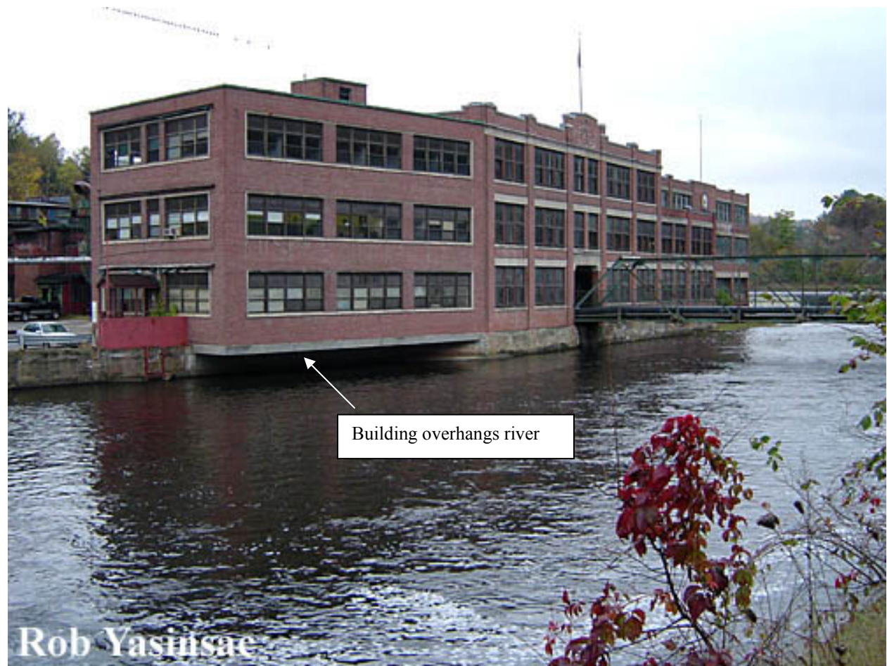
Figure 3-2. Photograph of main building from River Street. Used with permission from Rob Yasinsac / www.hudsonvalleyruins.org .
